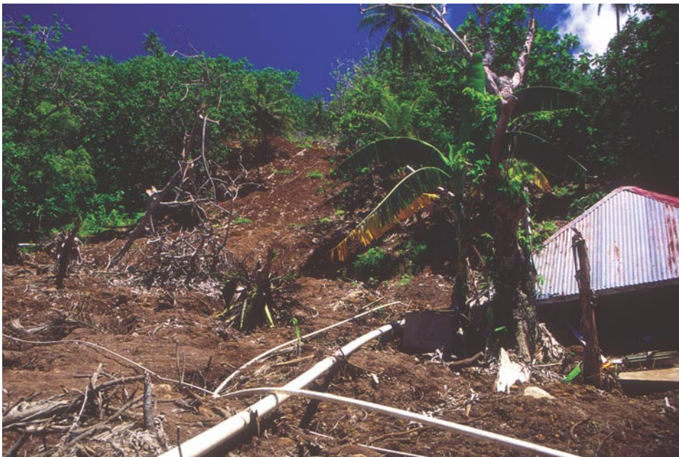
Figure 18. Lower portion of a slump/debris flow at the village of Sanuk on the island of Uman that destroyed 13 homes and a community center.
